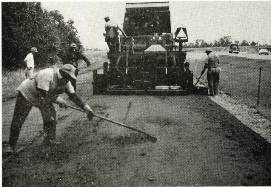
Large clumps in the mix caused some tearing in the mat. Constant hand raking was required to repair the mat.
