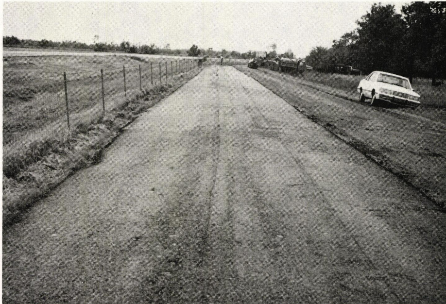
The freshly rolled mat seemed fairly tight with only a few segregated spots showing.
