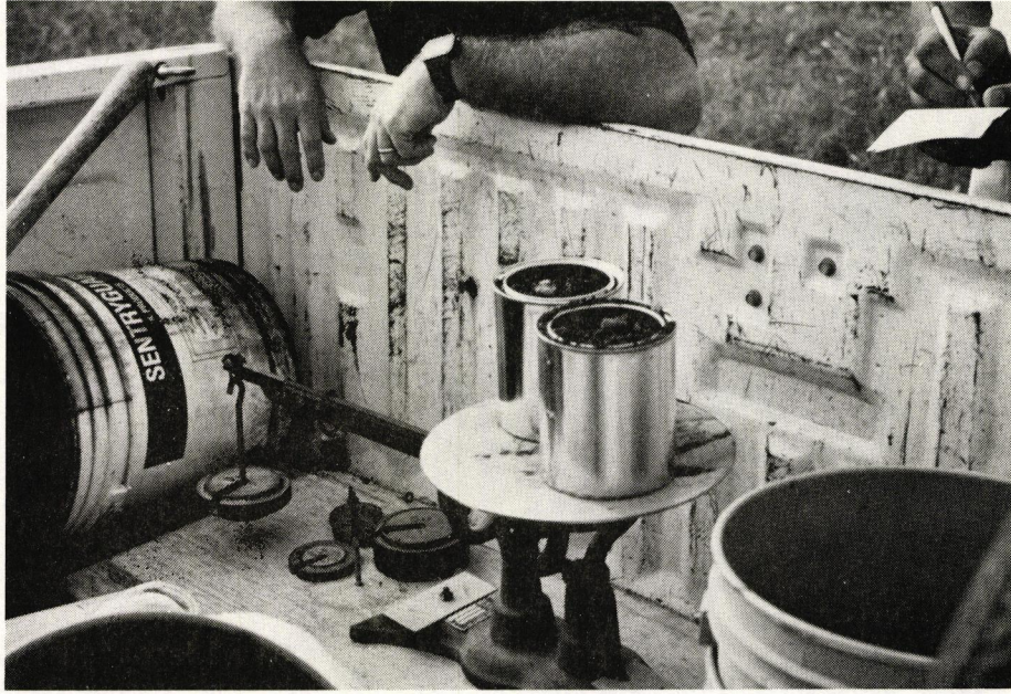
Samples of the mix were taken in the field to monitor moisture content and asphalt content.
